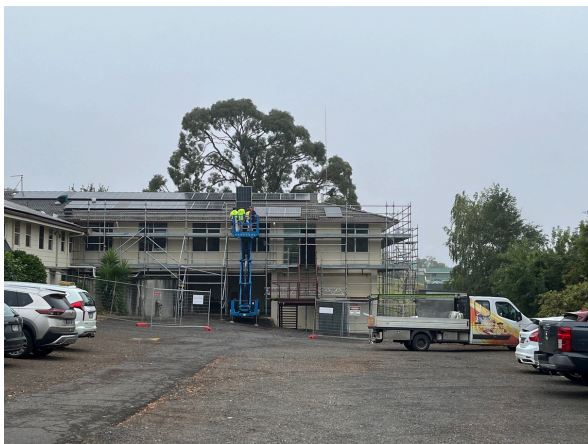
Solar panel removal.
